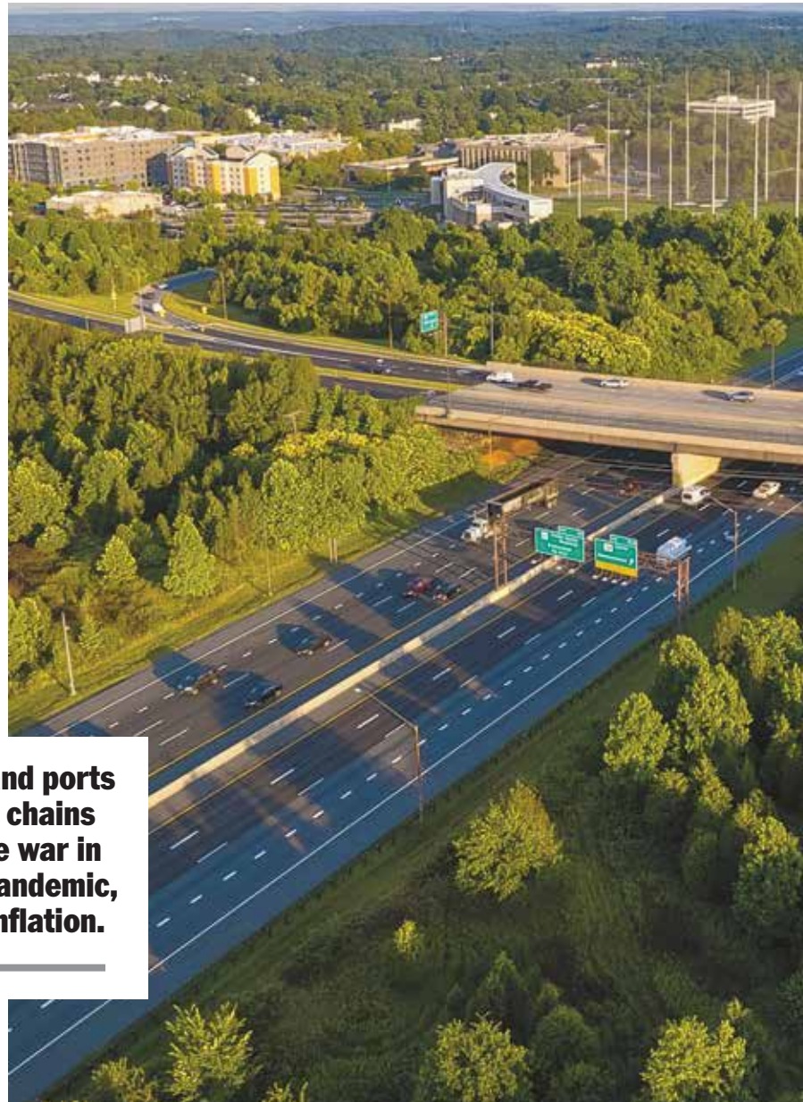
An aerial view of Dwight D. Eisenhower Highway near Germantown, Maryland.
