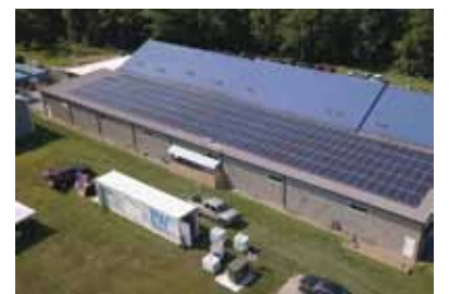
Behind-the-meter microgrid for load management and resiliency
