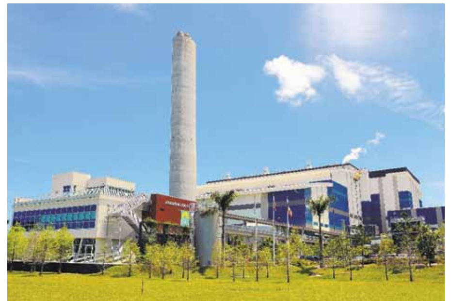
The Solid Waste Authority of Palm Beach County Renewable Energy Facility No. 2 is located in West Palm Beach, Florida. The plant processes up to 1 million tons of post-recycled municipal solid waste per year while producing enough power for 44,000 homes. Image courtesy of Babcock & Wilcox.
