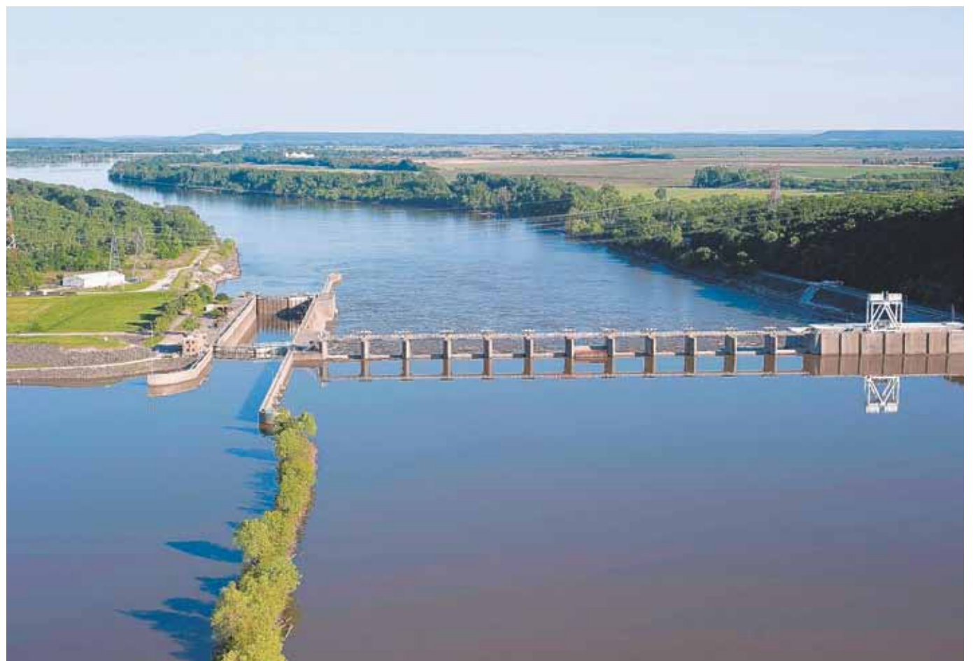
Webbers Falls Lock and Dam in eastern Oklahoma is one of 18 locks and dams in the 445-mile McClellan-Kerr Arkansas River Navigation System (MKARNS). The system supports agricultural and other commercial activity worth $3.5 billion a year. Photo courtesy of U.S. Army Corps of Engineers - Tulsa District.
