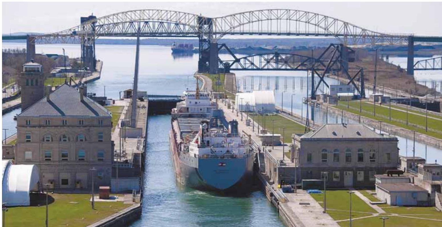
A ship navigates the Soo Locks between Lake Superior and Lake Huron on the St. Mary's River on United States (Michigan) and Canadian border. Image courtesy of the U.S. Army Corps of Engineers - Detroit District.
